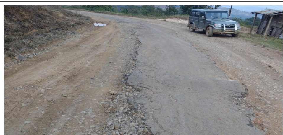
PHOTO: POOR ROAD CONDITION ON THE WAY TO SAIPUNG
